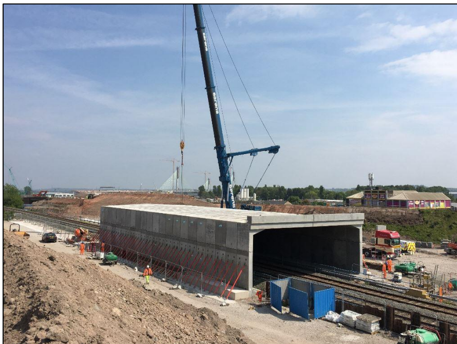
The new bridge over the Widnes deviation line was taking shape when this view was taken on 12 th May 2017. The bridge is part of the Mersey Gateway scheme and it is the only overbridge on the deviation line (the bridges that form part of the Silver Jubilee Bridge route being located at a point that was part of the original 1852 Warrington & Garston line). Photo courtesy of Merseylink
